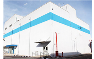
Mitsubishi Tanabe Indonesia Exterior view of new pharmaceutical production building
